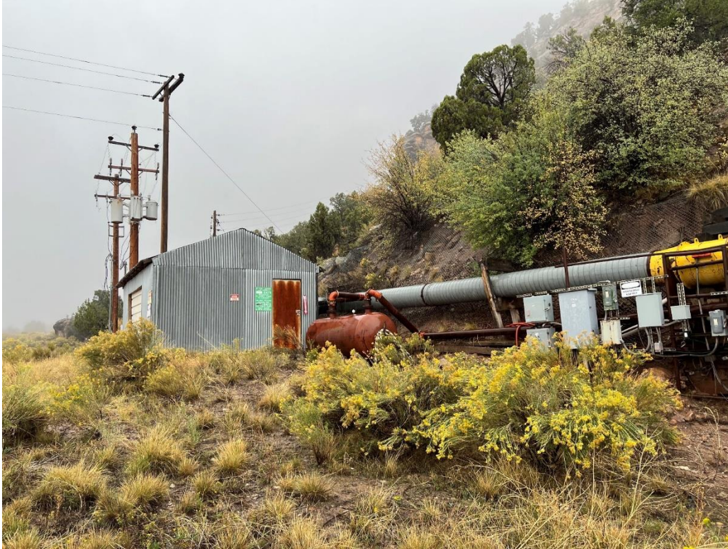
Figure 18: JD8 Underground Mine – Upper: power infrastructure and ventilation; Lower: adjacent mine portal
