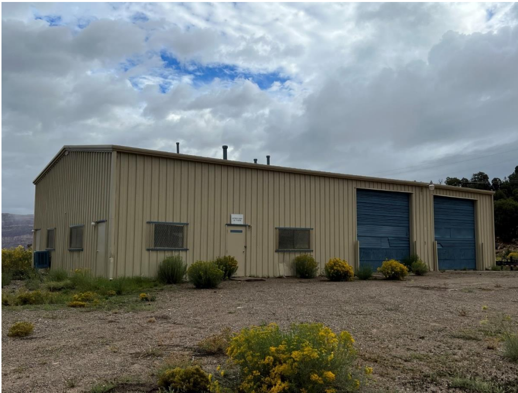
Figure 16: Upper: JD7 Mine support building; Lower: JD7 Mine rolling stock inside the shop
