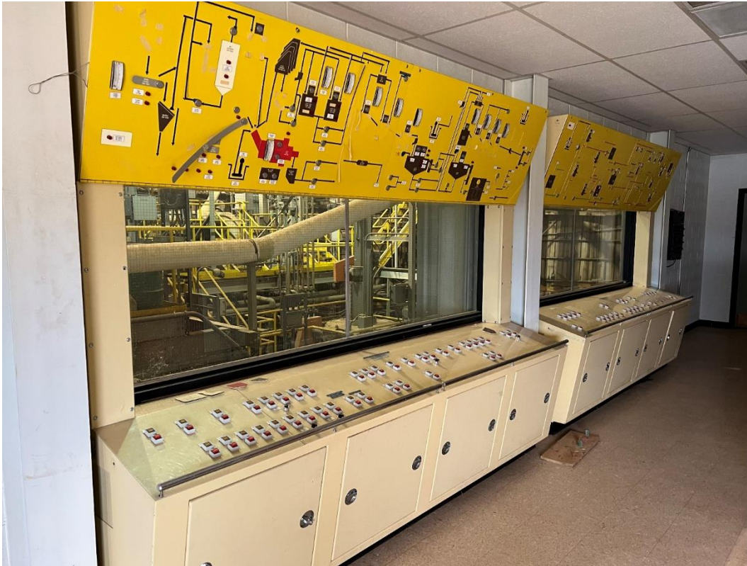
Figure 9: Upper/Lower: inside the control room at the mill – all of the systems controls will need to be modernized at refurbishment
